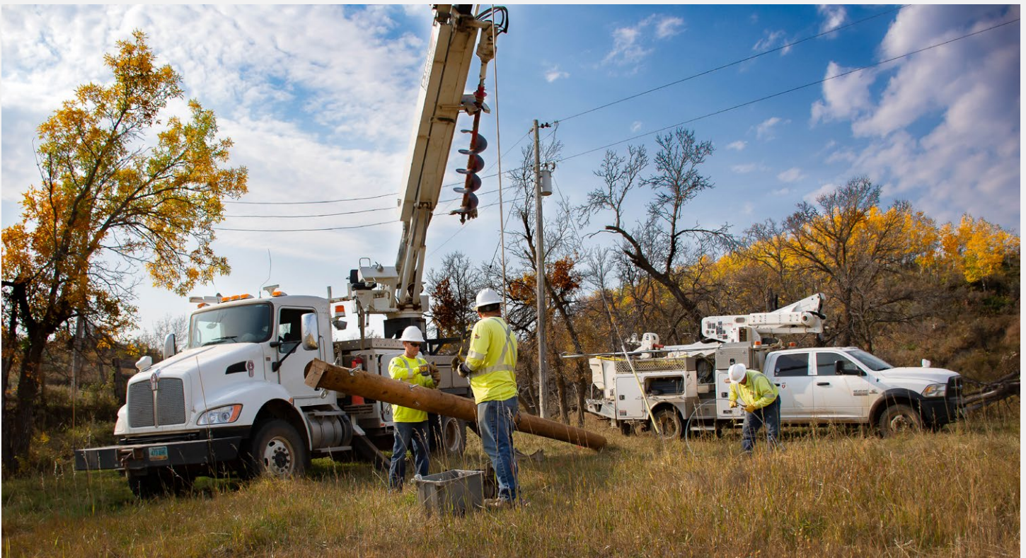
Roughrider Electric Cooperative's Dickinson crew including Journeyman Linemen Brock Swensrud, Mitch Krebs and Tyler Schlosser changing out a pole in the ND Badlands assuring reliable power supply to their member-owners. Photo courtesy of Roughrider.
