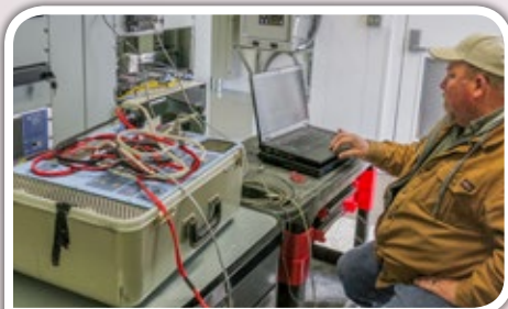
Chapman Metering technician conducting a meter test.
